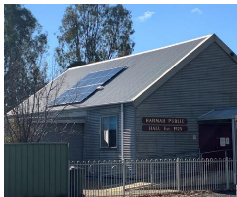
Image: New solar PV system at Barmah Community Hall (DELWP)
